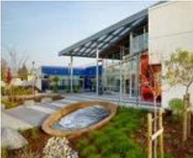
Fig. 7, Jackie Brookner, Chutes and Thumbprint Filter , 2008 Steel, pumice stone, rocks, sand, plants, wood chips, 16 x 13 x 6 ft, Roosevelt Community Center
