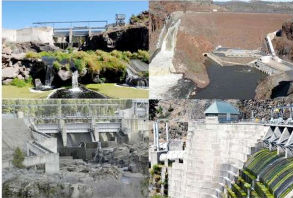
Figure 2. The four hydroelectric dams being considered for removal (clockwise starting in the upper right-hand corner) the John C. Boyle, the Iron Gate, and the Copco 1 and 2. 38
