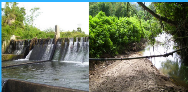
Concrete Dam of KMIS
